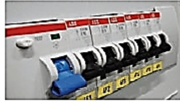
MCB - Miniature Circuit Breaker
