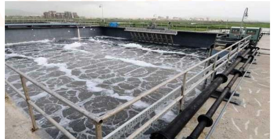
Figure 22.4 A view of sewage treatment plant
