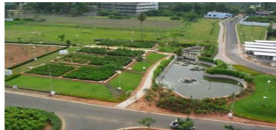
FIG. 12.6 (A) DEWATS SYSTEM AT AUROVILLE
